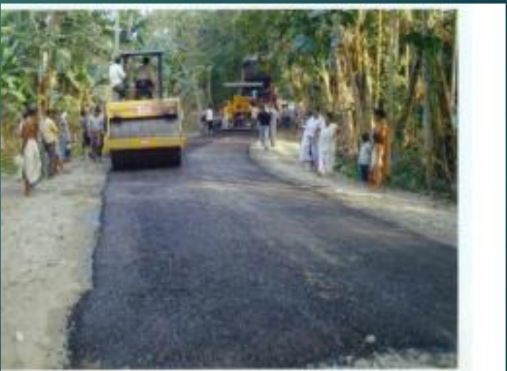
Rolling of Cold Mix
