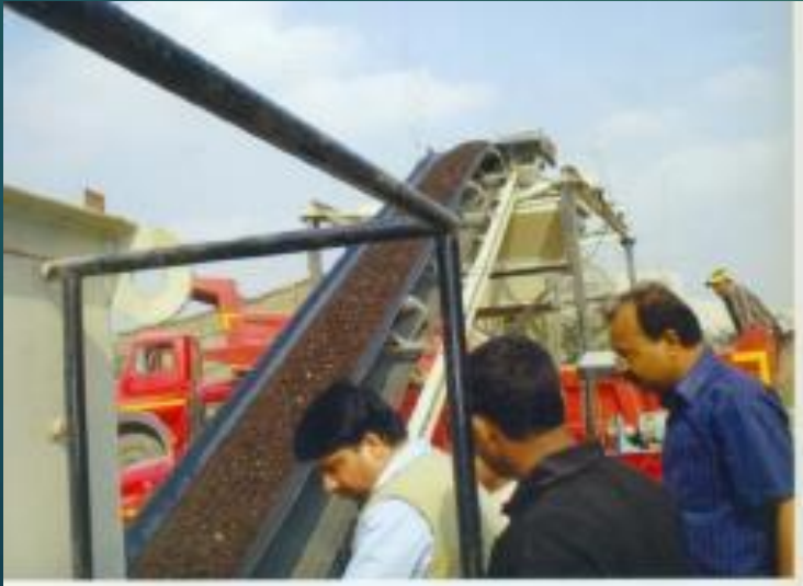
Preparation of Cold mix
